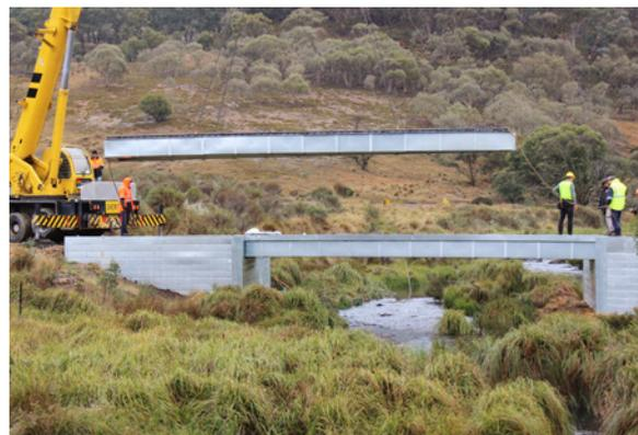
*Installation of the bridge panels onto standard InQuik modular abutments.*
