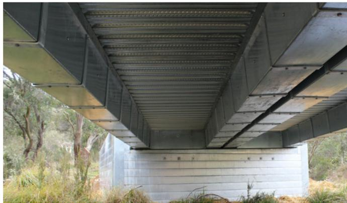
*View of beneath the InQuik deck panels, showing the integrated girders and deck.*
