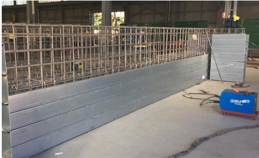
*An InQuik abutment in construction, showing the formwork and reinforcing components*
